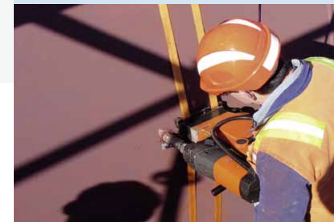
Drilling the sensor holes
